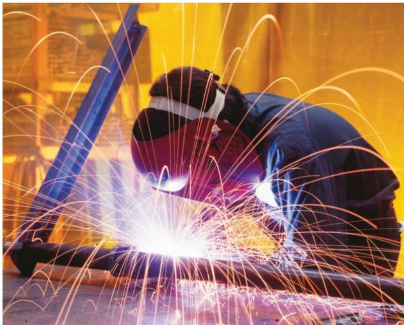
**Creating with Fire** The tremendous heat generated during welding softens a material until the parts can meld together. *Heat fastening only works with some materials. Why?*
